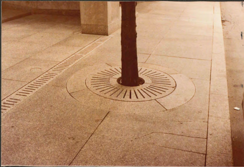
THESE TWO TREE GRATES USED IN TORONTO ARE AN EXPENSIVE, THOUGH ACCEPTABLE SOLUTION TO PIT COVERING IN THE SIDEWALK.
