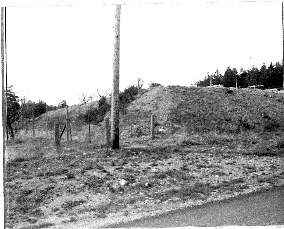
Steep Open Banks on the Southerly and Easterly Perimeter of the Station
