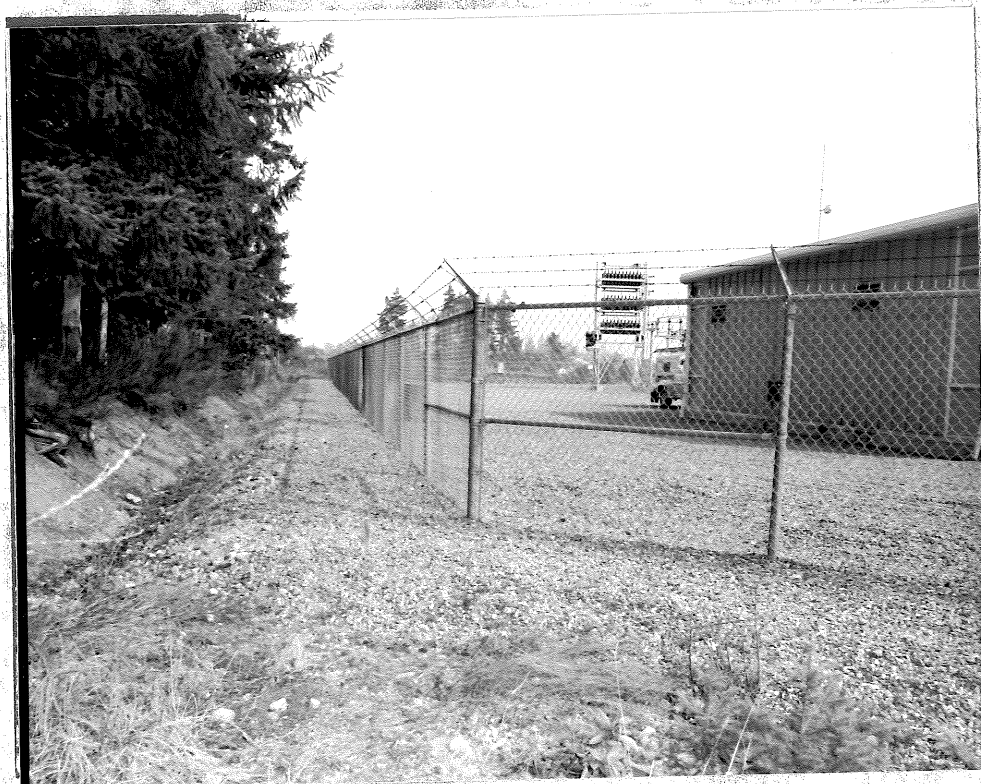
Shallow Catchment Drain on the North Boundary
