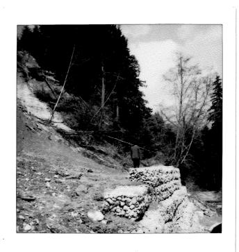
New clearing on Rabbit Lane has been followed by slumping now kept back by gabions. Little extra protection is afforded but the angle of repose for the lower slope may have been reached although it can be recharged from above.
