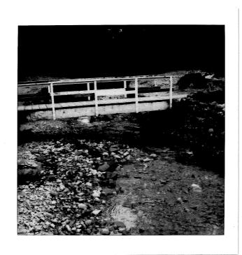
Bridge construction for property access intrudes into stream channel and will act as a partial dam at high flows. Design could be improved fairly simply.
