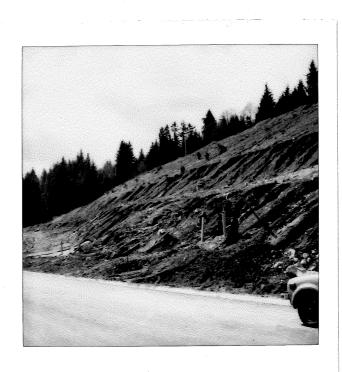
The extent of the cleared area at Rabbit Lane is evident as too are the many rills and gullies caused by surface water movement.
