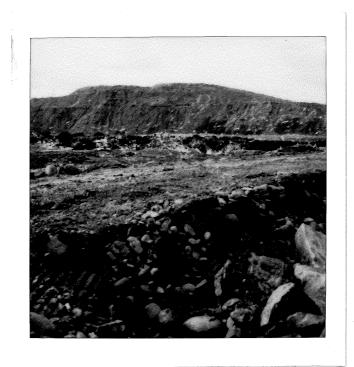
North Vancouver disposal site with new dyke in foregound, refuse to be covered in midground and depth of piling and covering to date in the background.
