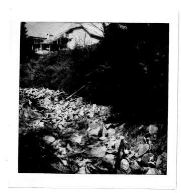
The support columns and wall for the swimming pool adjacent to this house are seen above Brothers Creek. Continued undercutting by the creek has been temporarily prevented by rechanneling and armoury of the creek bank particularly on the outside of the curve top left.
