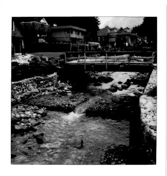
New gabion construction with cross-bar concentrator to ensure self-cleaning and to minimize stagnant water at low flows.
