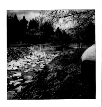
Outfall of lower Mosquito Creek tunnel shows wings, safety fence and energy dissipator. Stream banks are kept clean to provide unimpeded flow.
