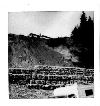
The proximity of housing to the edge on this silty terrace is becoming of concern particularly since no apparent measures have been made to protect the slope from erosion. New gullies can be seen caused by surface water from above.
