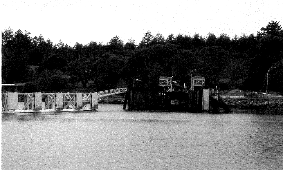
Texada ferry dock and ramp
